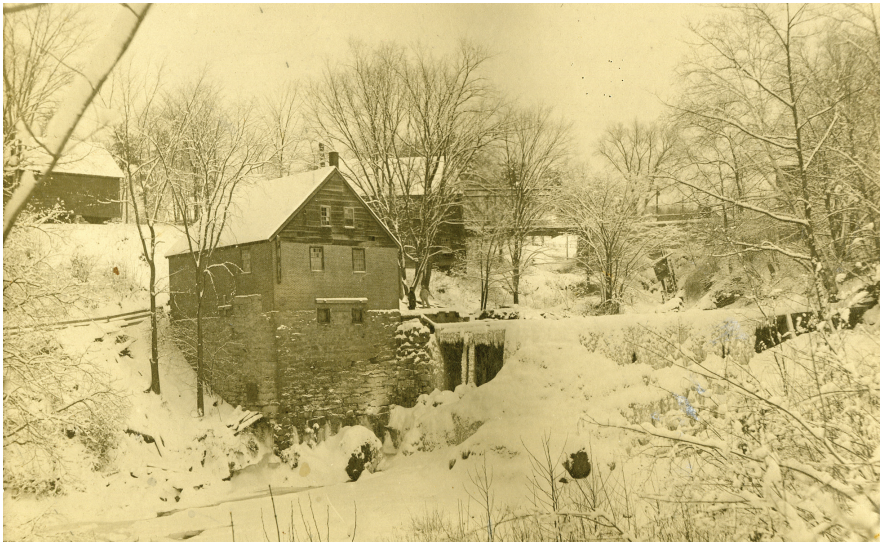
Photograph of Oliverian Falls, Haverhill, c. 1900 (left) and painting of the same scene (facing page) by Mary Lucinda (Hovey) Herbert (1828–1916), c. 1890. Thomas W. Slight purchased this grist mill in 1898 and operated it until it was destroyed by a flood in 1927. The two items were donated to the Society in 2015 by Elizabeth Oatley, a descendent of Slight.
